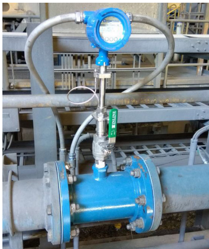
Fox Thermal model FT4A thermal mass flow meter and temperature transmitter.
